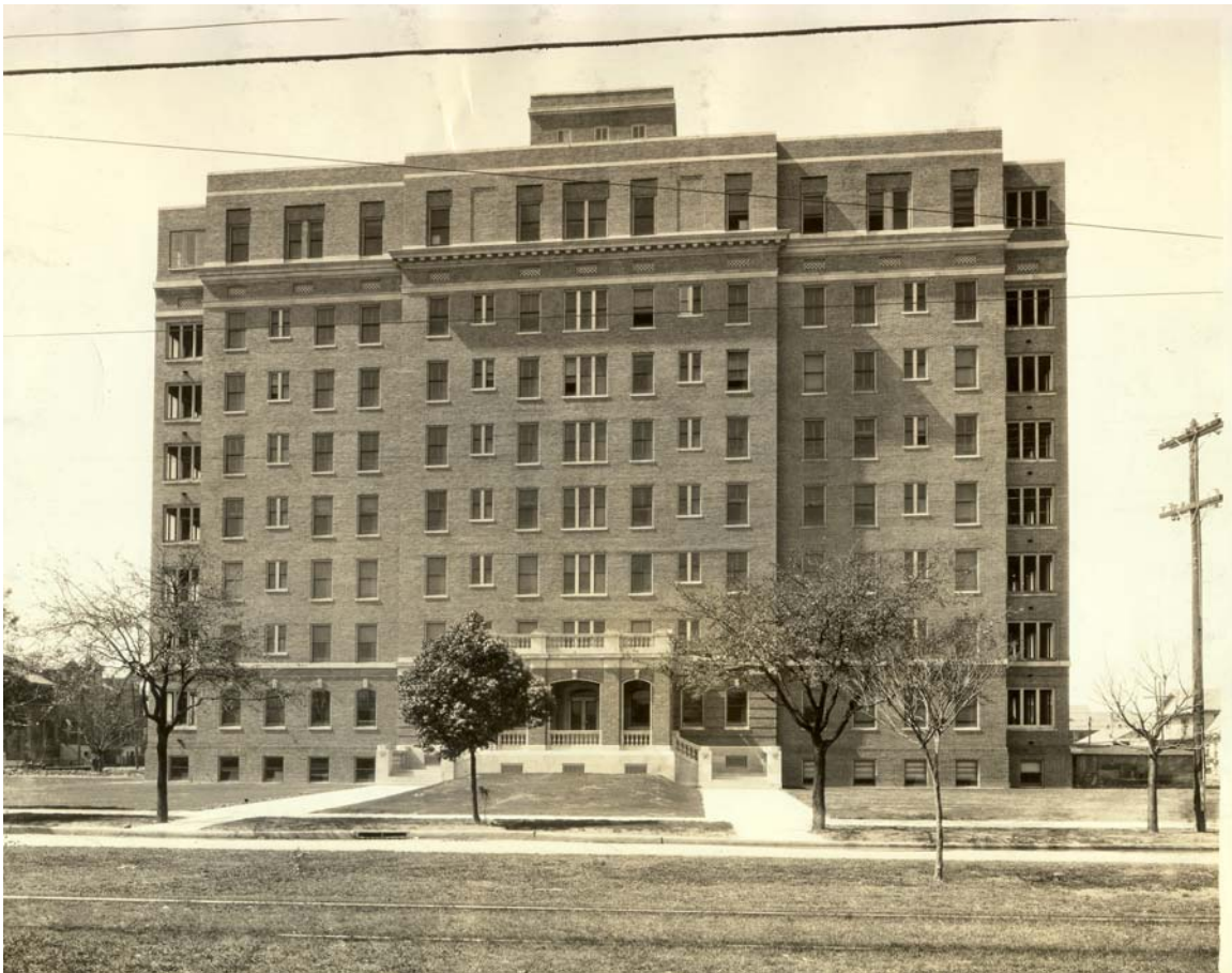
Southern Baptist Hospital, New Orleans, Louisiana, c. 1945
